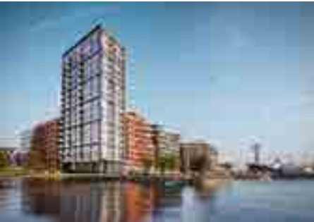
South Dock Amsterdam
